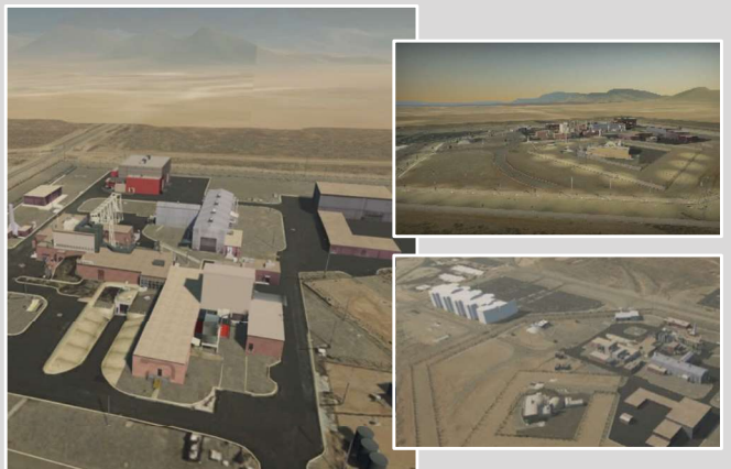
Springfield Processing Facility Cat I
